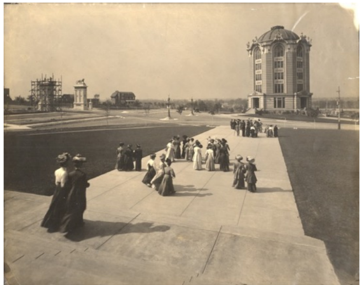
Above: Sixty-five women, almost all members of the American Woman's League, from Edwardsville and East St. Louis, Illinois visited University City and League headquarters on May 7, 1909. On the left, the Lion Gates are under construction. One is complete and the lion has been installed. The other pylon is still surrounded by scaffolding. This photograph appeared in "The Woman's National Daily" on May 10, 1909. (From the University City Public Library Collection.)
